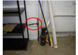
Marginal Water Lines: Galvanized and copper - Copper to galvanized supply piping connections lacks dielectric unions
