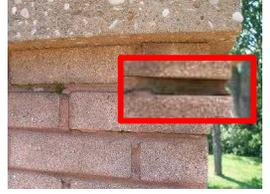
Defective Flue/Flue Cap: Concrete - **Noted crack(s) in crown**
