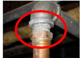
Marginal Drain Pipes: Galvanized, Cast iron - Galvanized drainpipe present, Galvanized piping is subject to corrosion and will eventually require updating
