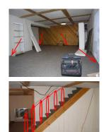
Defective Basement Stairs/Railings: Wood stairs with no handrails
